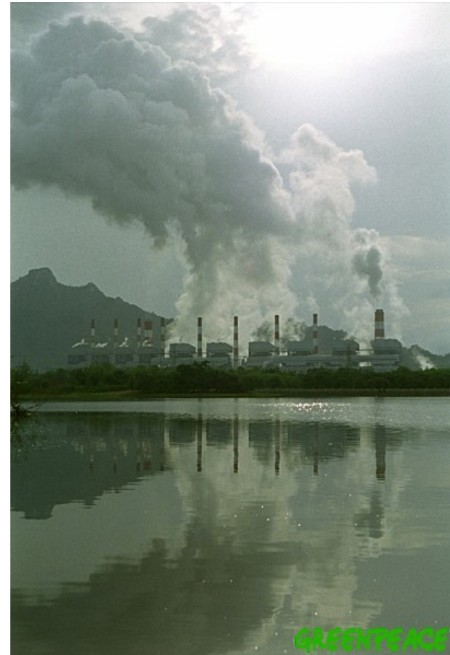
Coal power plant in Thailand
